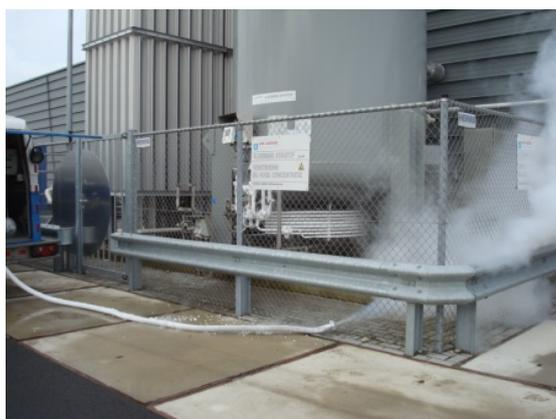
*Figure 5 Source of Liquid Nitrogen for Gas Conversion*
